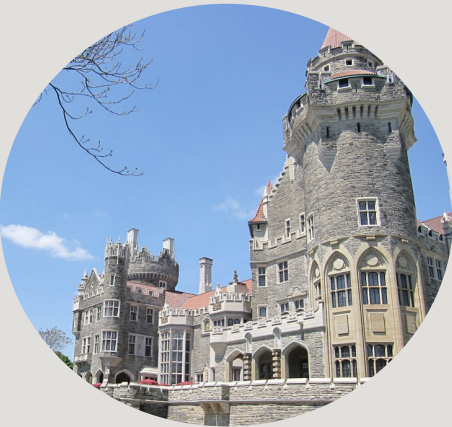
Casa Loma 1 Austin Terrace
